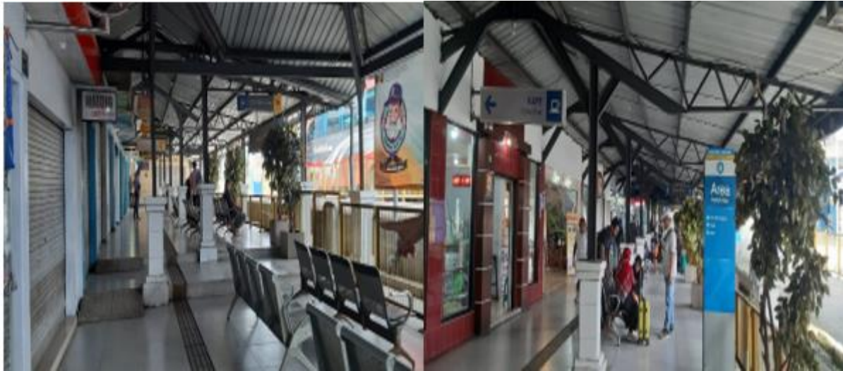
Figure 2. Arjosari Malang Bus Terminal: Waiting Area
