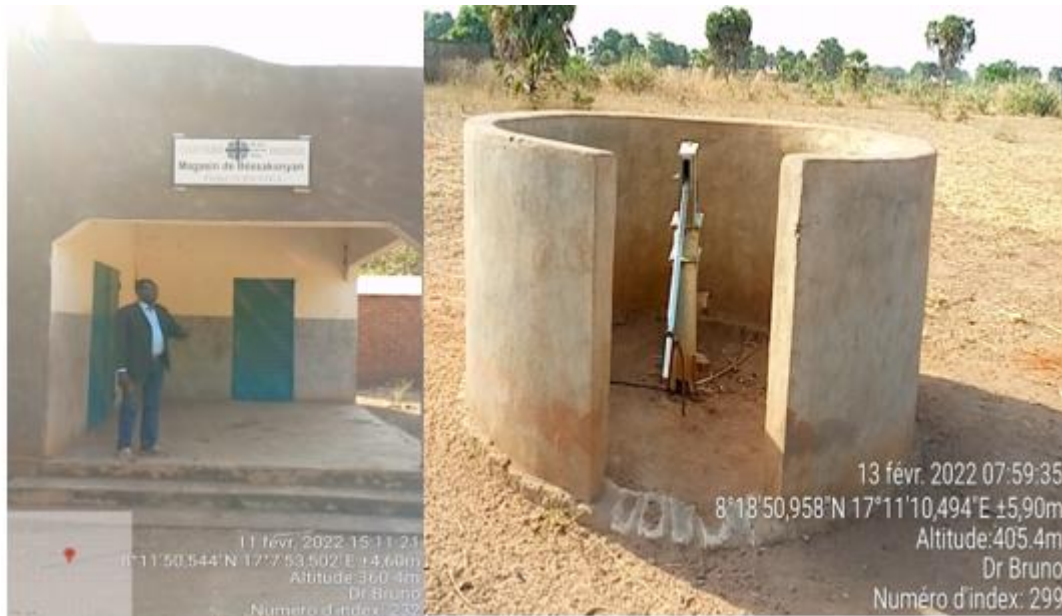
The photo on the right shows the Bèssakonyan store, built with financial support from SODEFIKA (Support for the shea and peanut sectors) and the photo on the left shows a human-powered drilling operation in Békonda.
